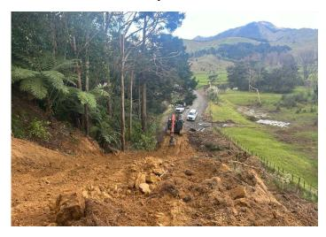
Slip-prone hillsides are being benched which involves flattening areas above and/or below the roads to provide a stable base for fill.
